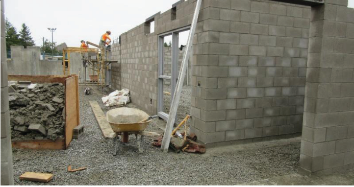
Walls being built in the Parish Hall.
